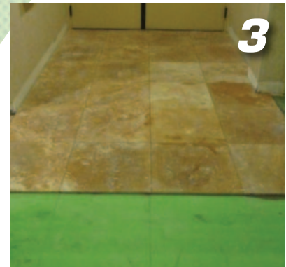
3 Lay Thinset and Flooring Directly on GreenSkin™
