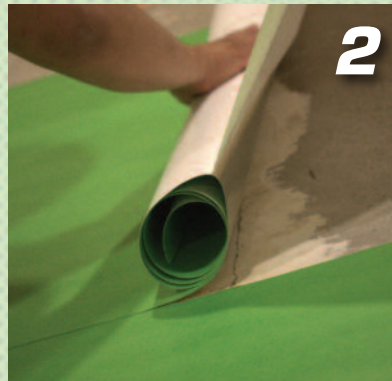
2 Remove Backing and GreenSkin™ Adheres Directly to Substrate
